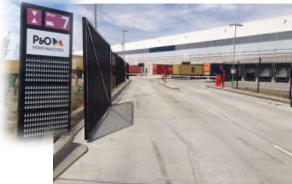
Site entrance – West 7
