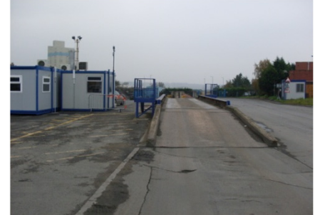
EXIT VIA WEIGHBRIDGE AND GATE A
