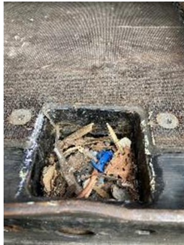
Chalk line shows 3cm max depth post was seated
